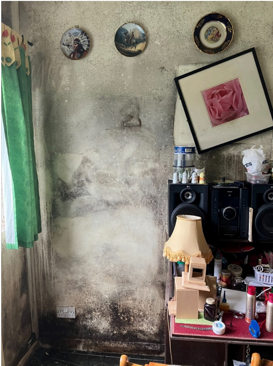
Black mould in the house of a disabled Thirteen tenant in Billingham
